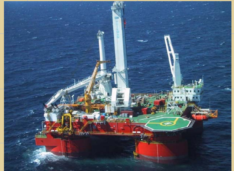
Q-4000 – Jumper Installation
