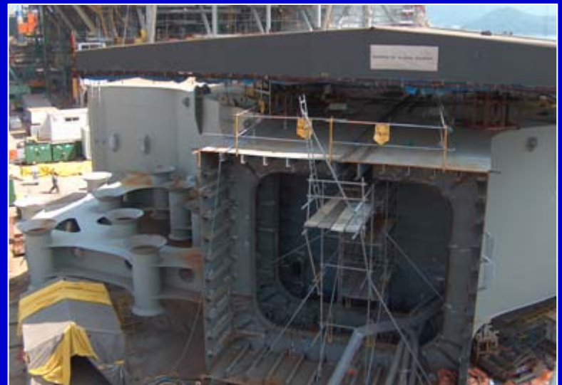
Oveng BS showing well slots
