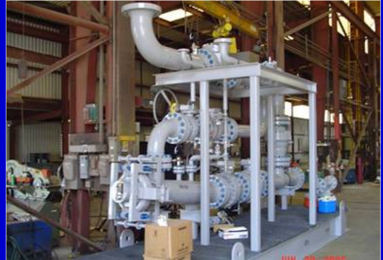
Pig Launcher Skid Fabrication
