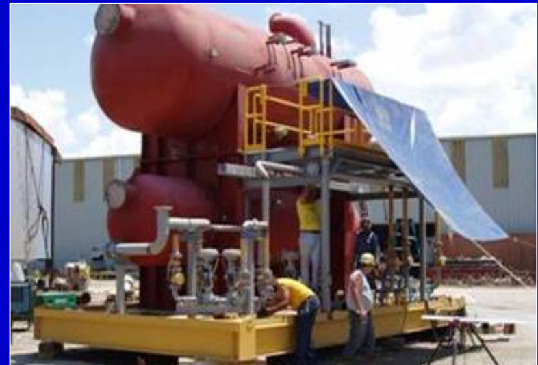
Production Skid Fabrication
