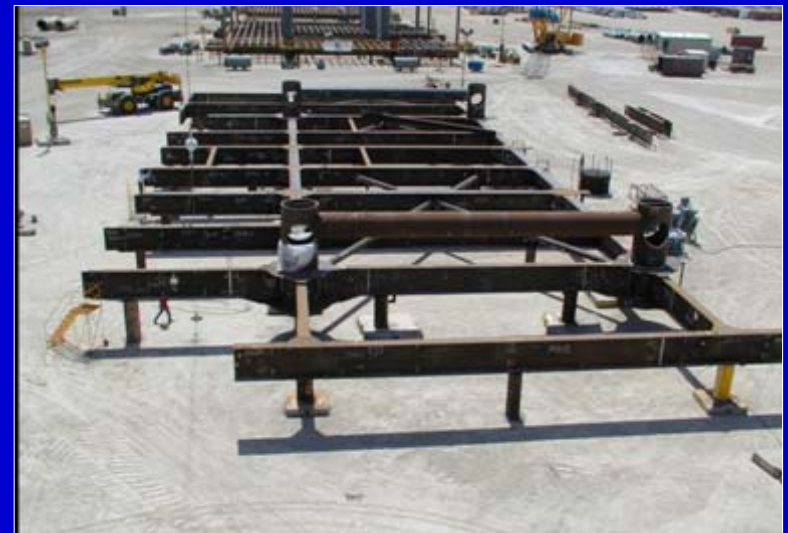
CPF main deck framing
