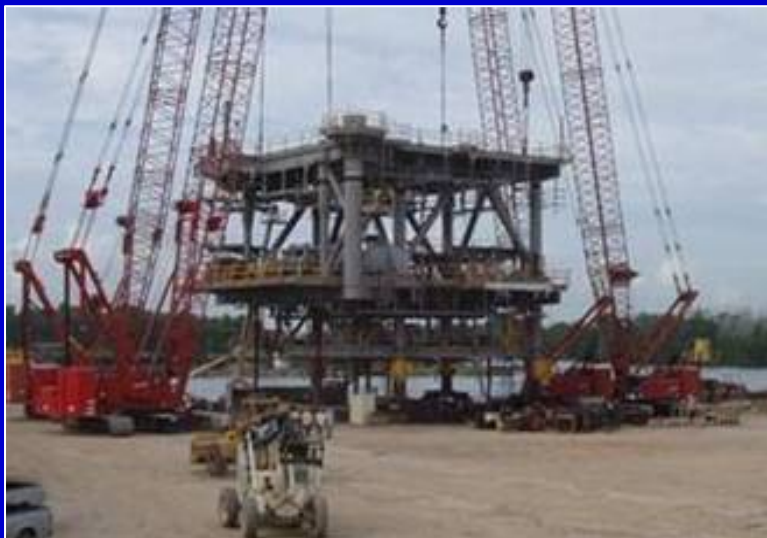
Main deck float – Sat. 2
