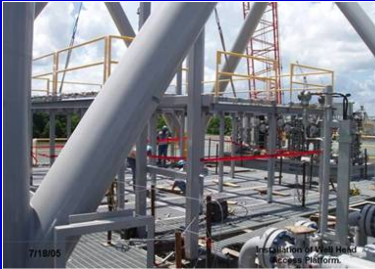
Installation of Well Head Access Platform
