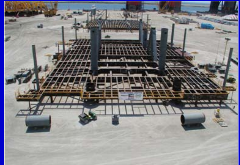
CPF cellar deck framing
